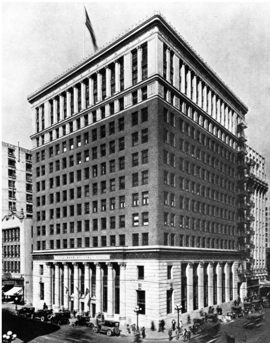
Figure 1: Bank of Italy Building, corner view. Undated. Source: Security Pacific National Bank Collection, Los Angeles Public Library Photo Collection.
